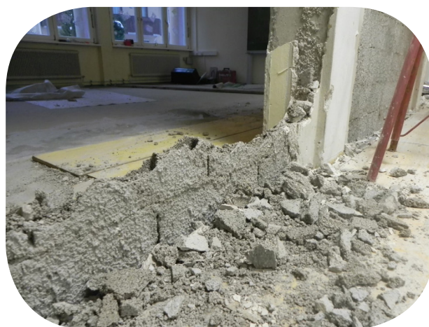
Breaking down walls, Zell am See School, Austria
